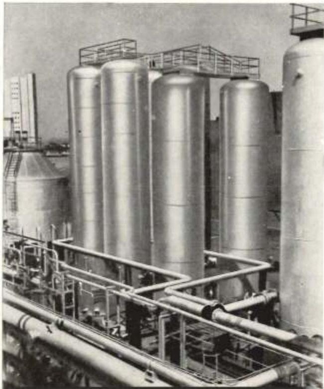
100 m 3 Gaseous oxygen vessels designed to ASME Section VIII Division 2 for a pressure of 34 kg./cm 2 g.
