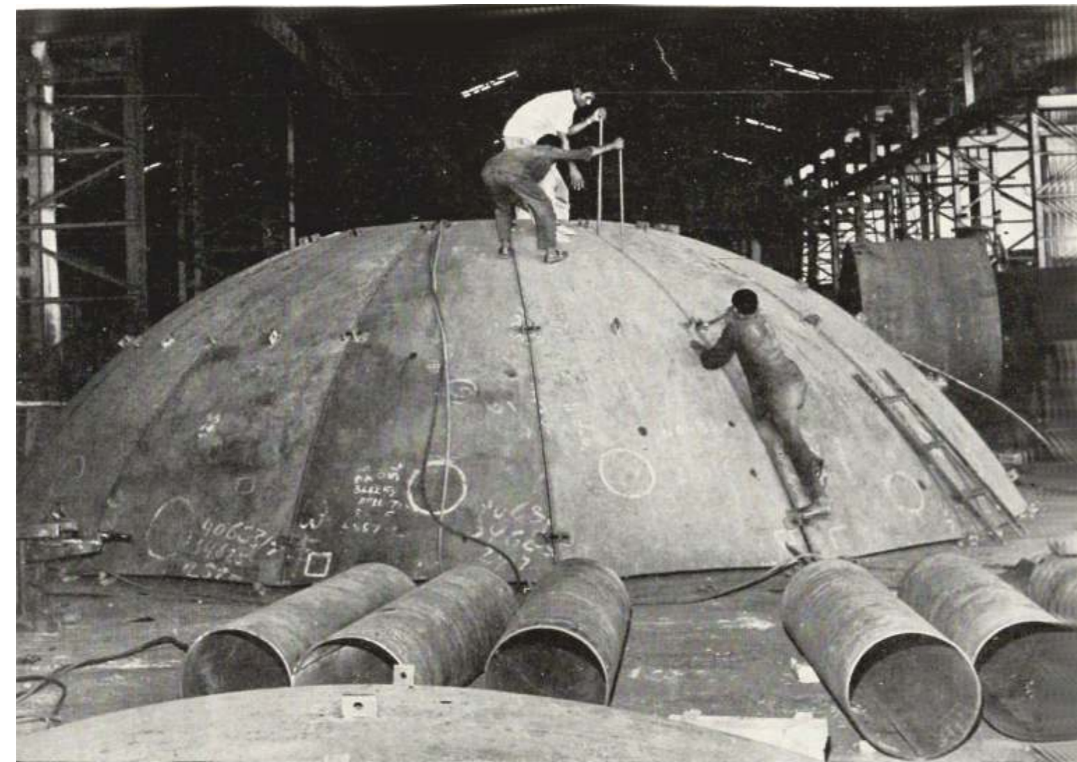
Mock fit-up of sphere petals in progress at shop
